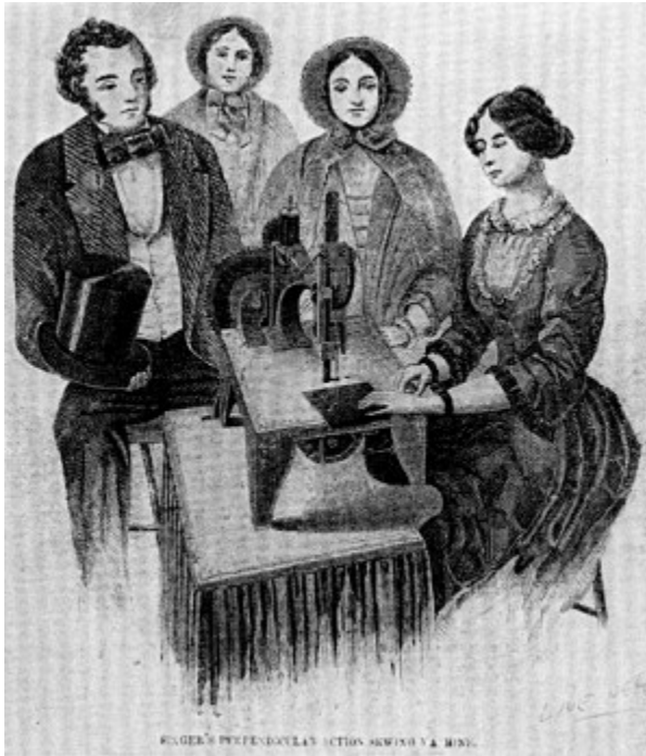
Figure 29.—SINGER’S PERPENDICULAR ACTION sewing machine, an engraving from Illustrated News , June 25, 1853, which states: “The sewing machine has, within the last two years acquired a wide celebrity, and established its character as one of the most efficient labor saving instruments ever introduced to public notice.... We must not forget to call attention to the fact that this instrument is peculiarly calculated for female
