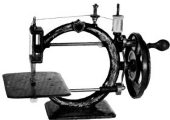
Figure 73.—BARTLETT SEWING MACHINE, 1867. The Bartlett machine was first manufactured in 1866 under the January 31, 1865, and October 10, 1865, patents of Joseph W. Bartlett. The machines were made by Goodspeed & Wyman for the Bartlett Co. and were so marked. The inventor received another patent on April 7, 1868, and later machines carry this third date
