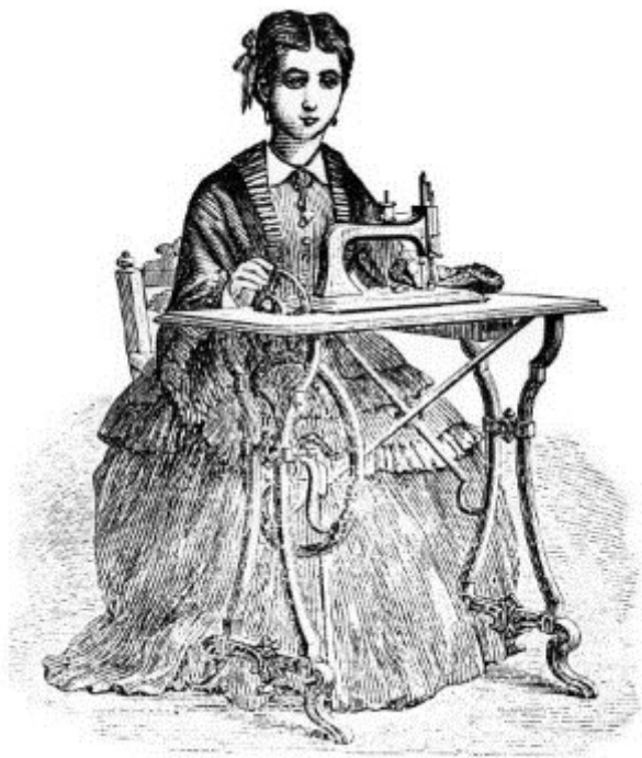
Figure 92.—GROVER AND BAKER SEWING MACHINE. The Grover and Baker machine was one of the more popular machines from the 1850s until the early 1870s. The company produced iron-frame machines, fine cabinet models, and portables (figs. 35
